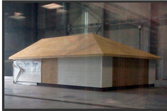
Premature siding loss due to lack of proper siding installation (missing fastener at lap joints) as investigated in a full-scale wind tunnel facility. Source: Institute for Business and Home Safety
