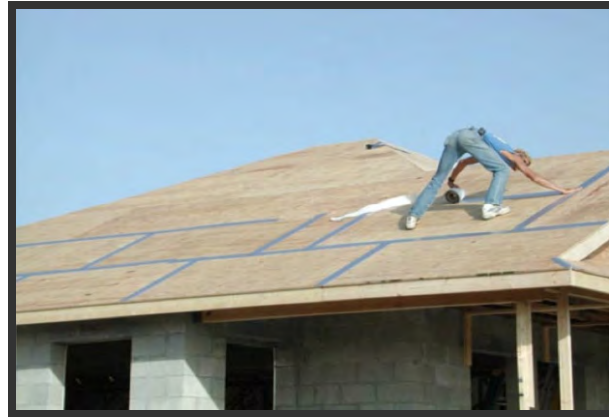
Bituminous ‘peel-and-stick’ flashing tape applied to roof sheathing joints. Photo Source: Institute for Business and Home Safety.
