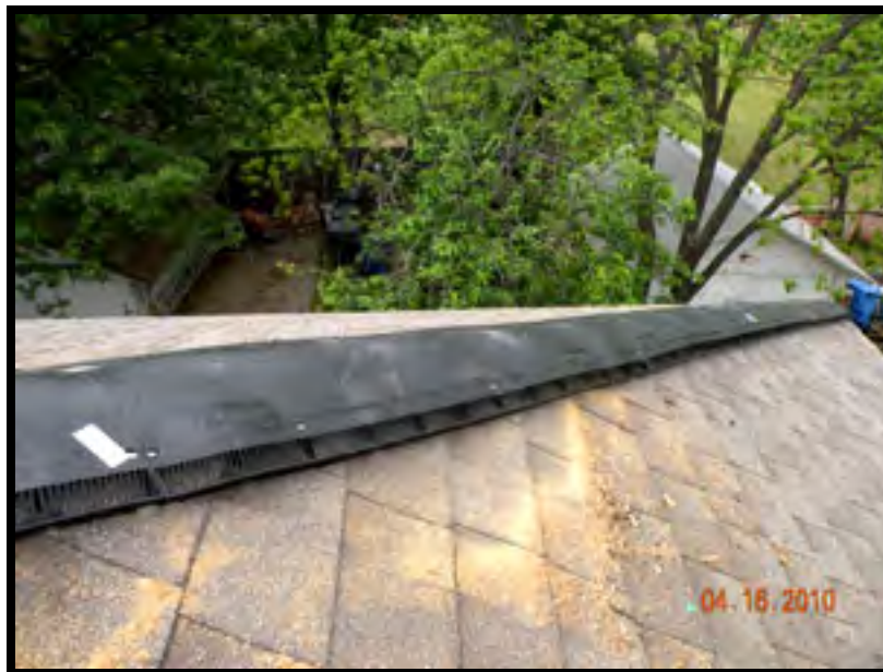
Example of a shingle-over vent with baffles to resist water entry. This product has a listing with the Texas Department of Insurance. Used with permission from Hip Ridge Vent by Air Vent, Inc.
