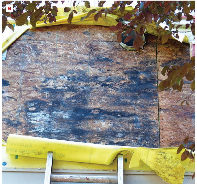
On a multifamily housing complex in Washington state, removal of contact-applied vinyl siding, paper, and gypsum sheathing revealed moldy, decayed OSB (5). The damage was worse on the inside face of the OSB. On a different housing complex in Oregon (6), moisture driven from the interior caused sporadic deterioration of the WRB and decay of OSB sheathing.
