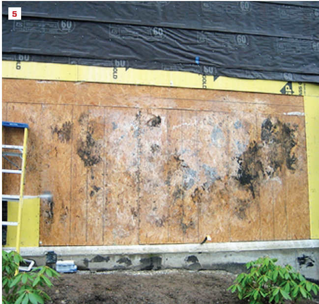
On a multifamily housing complex in Washington state, removal of contact-applied vinyl siding, paper, and gypsum sheathing revealed moldy, decayed OSB (5). The damage was worse on the inside face of the OSB. On a different housing complex in Oregon (6), moisture driven from the interior caused sporadic deterioration of the WRB and decay of OSB sheathing.
