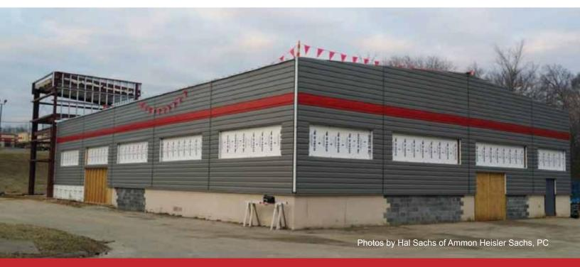
InsulWall R-Tech was used as the exterior wall insulation for the building's metal wall panel system.
