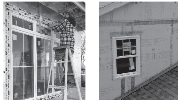
■ Figure 4. FPIS WRB System installation using joint tapes and adhered flashings; refer to manufacturer installation instructions for specific details.
