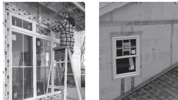
Figure 4. FPIS WRB System installation using joint tapes and adhered flashings; refer to manufacturer installation instructions for specific details.
