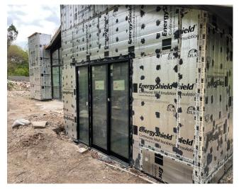
"The foil facer on EnergyShield makes a significant difference in the energy performance and heat resistance of the house," said Petrini. "Before we installed the siding and just had the EnergyShield exposed, you could feel the heat radiating off it. So, to see and feel the heat radiating off the insulation demonstrated so much of the effectiveness of the product because we knew it wasn't going into the home." Petrini was immediately confident in his decision to choose Atlas EnergyShield.
