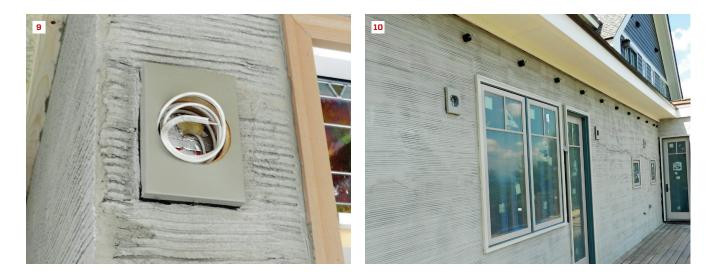
The mason applied a very heavy scratch coat to provide a secure bond for the stone veneer. For the mortar, he used Spec Mix Stone Veneer Mortar VM-01 (9). The entire first floor below the second-story beltline was stuccoed, including above the rear deck (10). Note: The standouts just below the soffit are for a ledger board that will support a trellis. With any cladding material, especially one like stone that can hold a considerable amount of water, it's important to promote drainage and drying.
