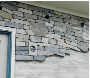
By the end of the project, everyone involved was a convert to the idea that real veneer stone could be successfully installed on top of relatively thick foam. The clients are extremely happy with the way the stone looks after three and a half years (15). There are no indications of any cracking, none of the stone has come off, and the exterior surface is selfcleaning when it is rained on, so it still looks quite good.
