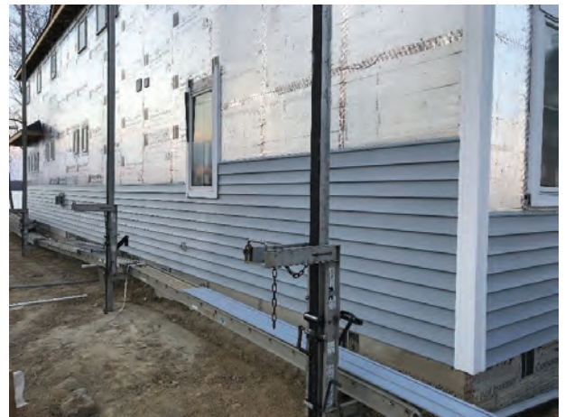
Photo 2. Code-compliant installations of vinyl siding over FPIS ci.
